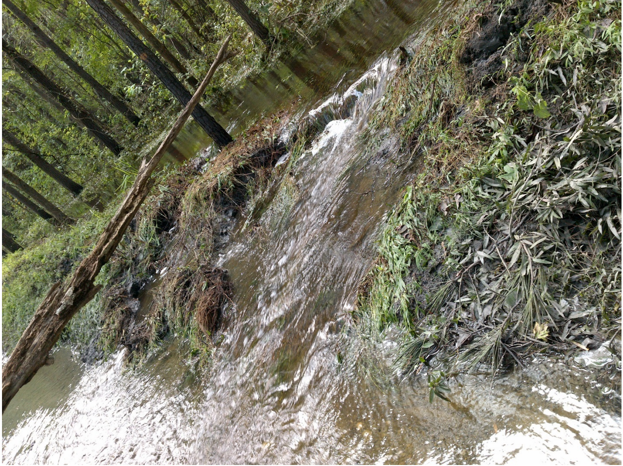
Flowing floodwaters exiting ash basin across basin dike wall.
