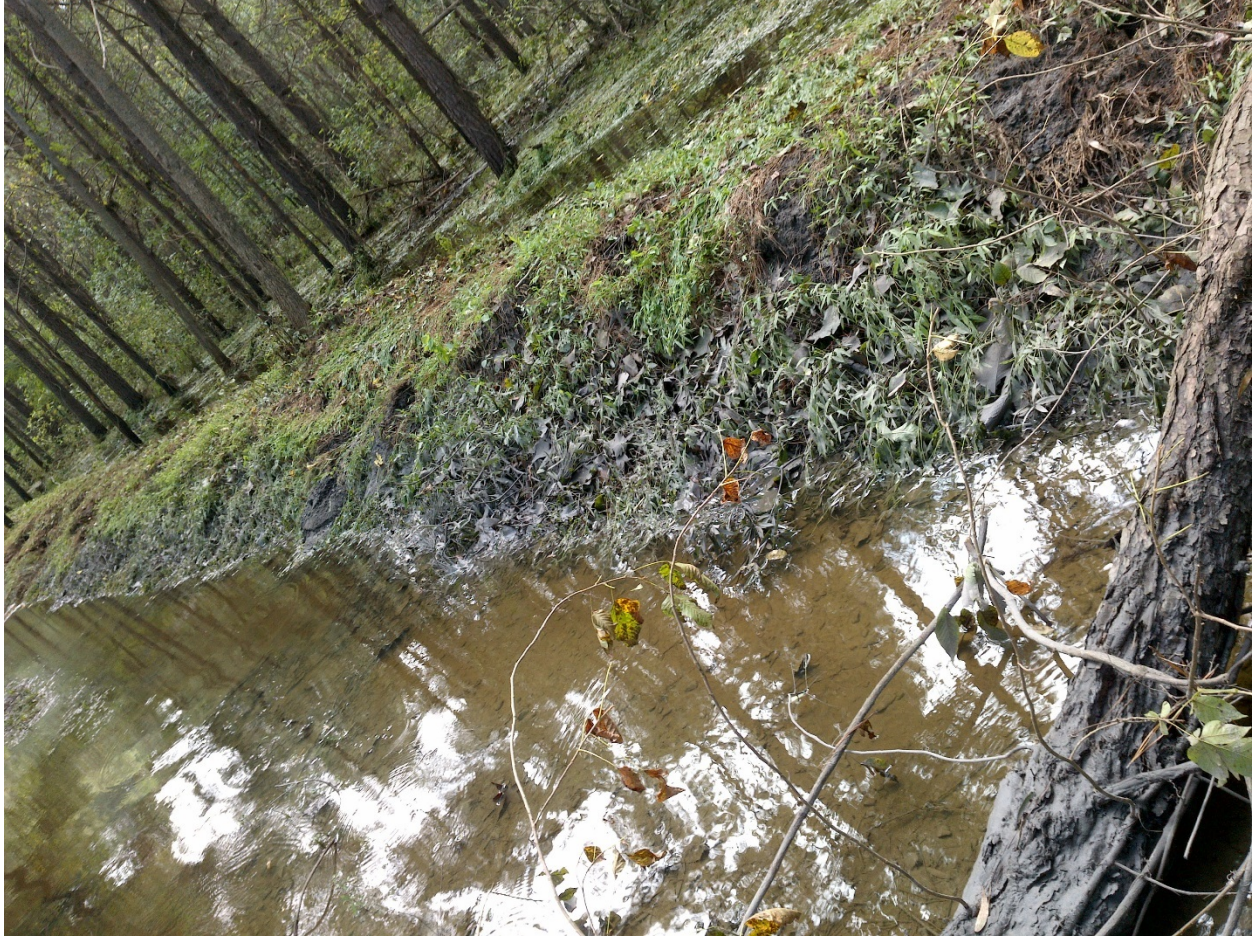
Flooded ash basin complex behind dike wall boundary. Some silting/ash along outside of ash basin dike wall.
