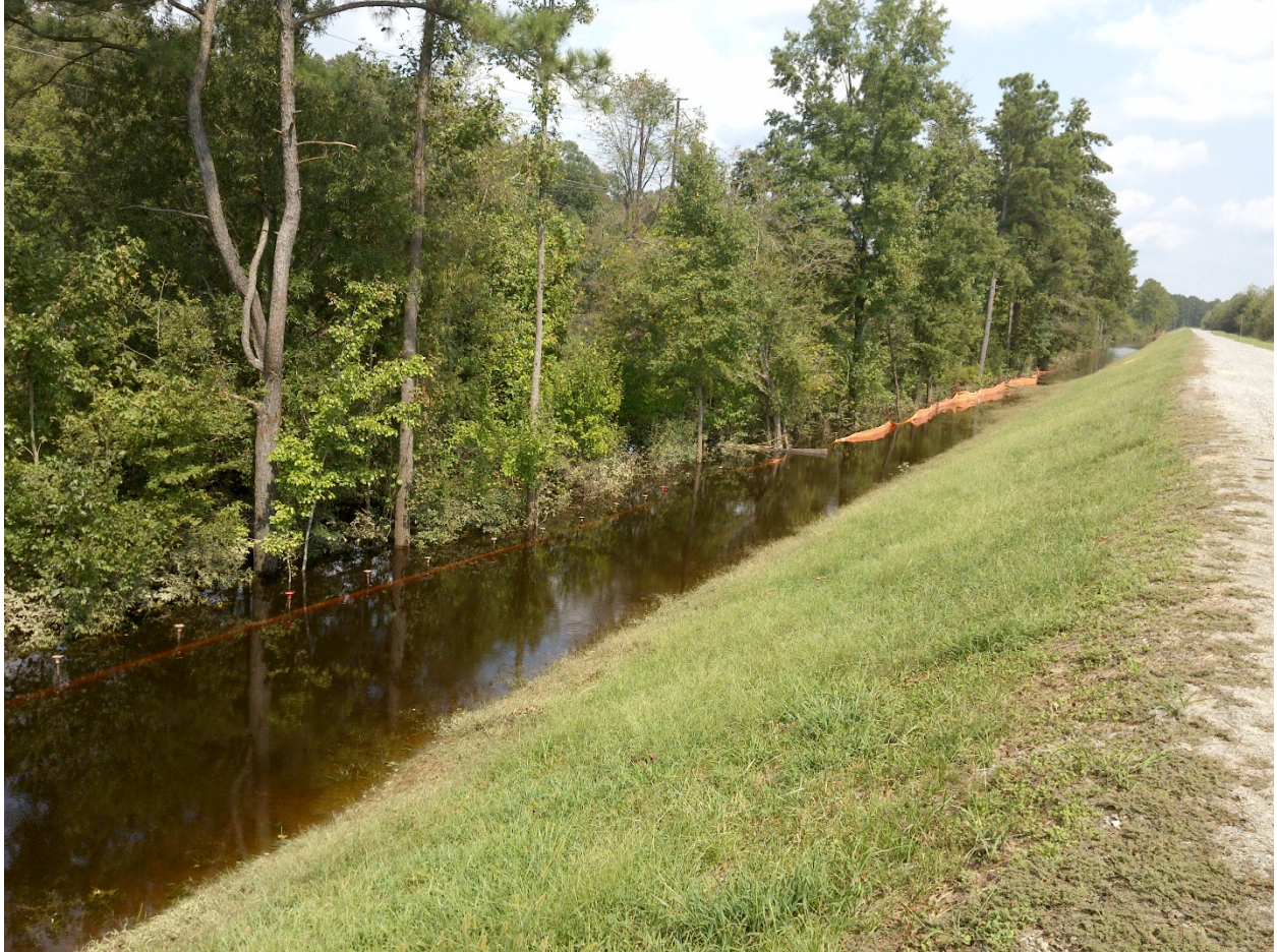
Neuse River floodwaters encroaching on active ash basin dike wall.
