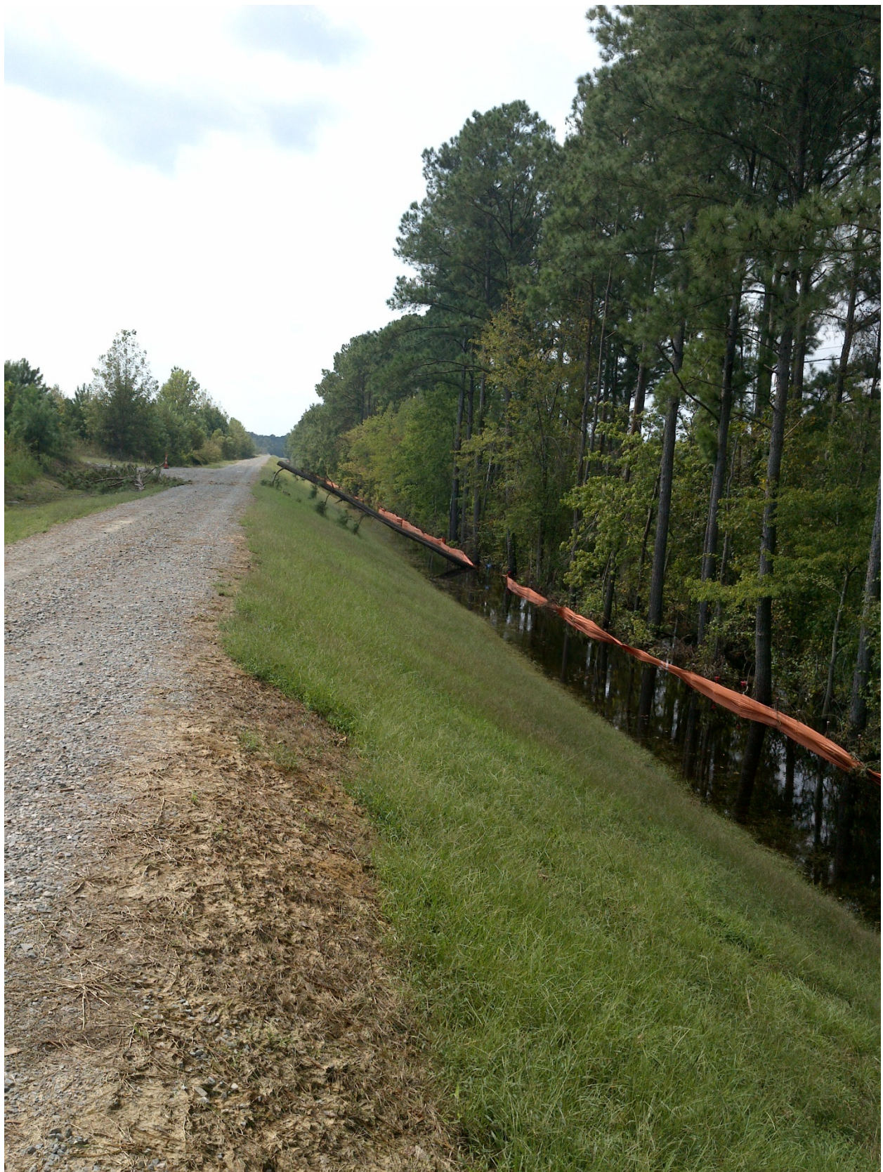
Neuse River floodwaters encroaching on active ash basin dike wall.
