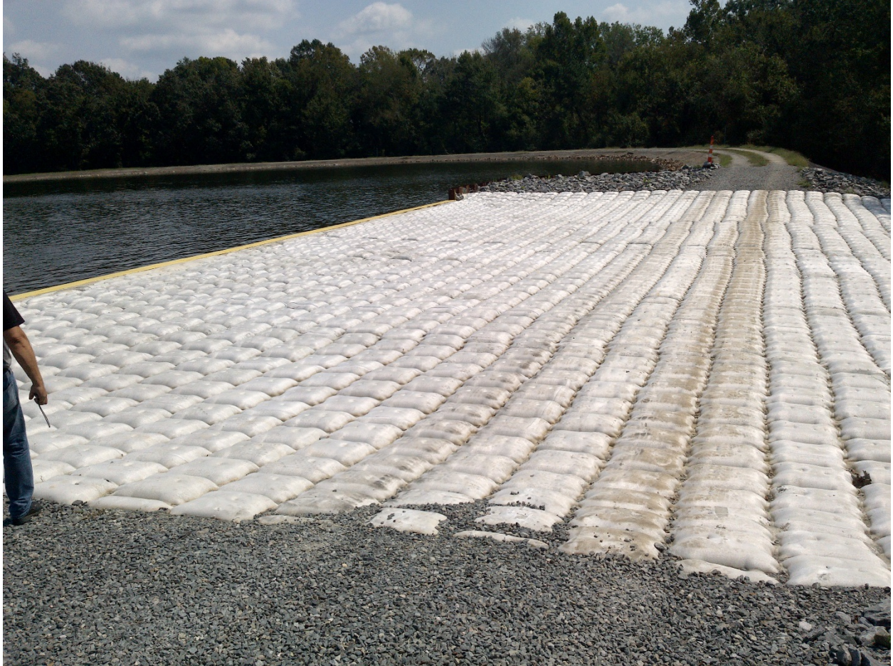
Newly constructed cooling pond emergency spillway.
